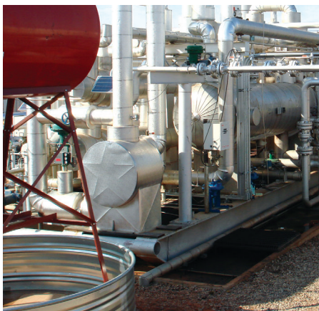
Compact, skid-mounted propane condenser.
