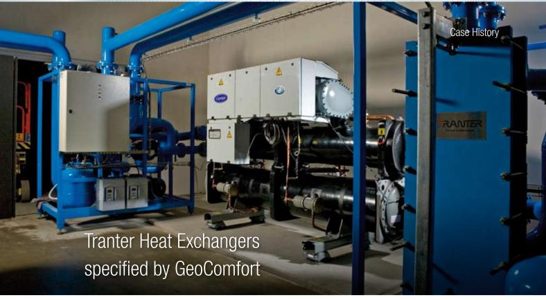
Tranter has been contracted to deliver heat exchange components for use on all of GeoComfort standard geothermal products.
